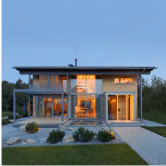
Bio-Effizienzhaus Alpenchic, Deutschland, Poing "Alpenchic" renewable energy-efficient house in Poing, Germany
